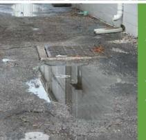
**Grade Depressions:** Areas of high traffic (wherein heavier equipment or vehicles are used), or exposure to large amounts of standing water contribute to grade depressions in your pavement. Grade depressions are localized and are indicated by low depressions on the surface of your pavement.
