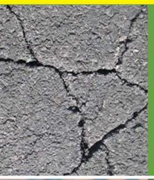
**Cracks:** Asphalt cracks have many names and causes. Types of cracks include: shrinkage, longitudinal, reflection, alligator, interconnecting, or any cracks parallel and evenly spaced along the surface of your pavement. Causes of cracks vary and are caused by erosion, unstable conditions of the ground, oxidation (which contributes to shrinkage), weakened/weathered joints, and fluctuation in temperature are just a few of the culprits creating cracks in your asphalt.
